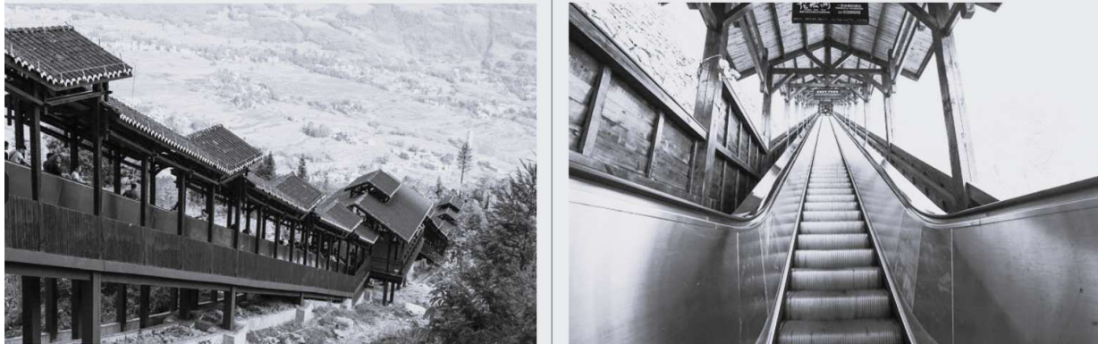
Figure 3 Escalators inside Tunnel in Outdoor Environment. (Williams, 2016)
